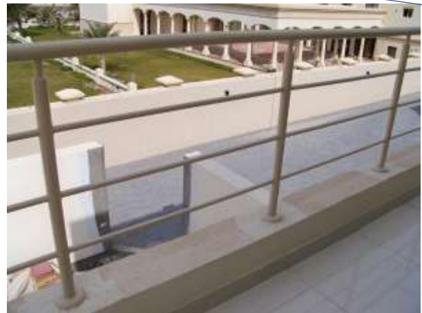
Painted steel balcony railing
