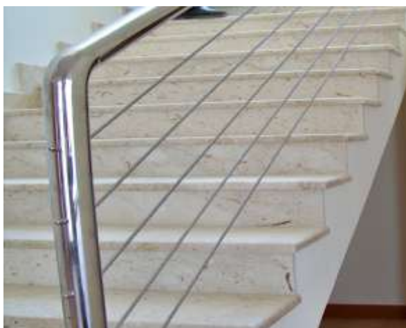
Stainless steel wire rope railing
