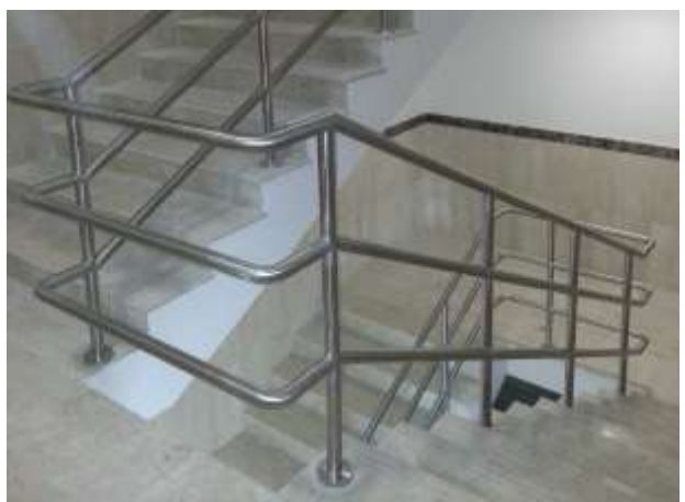
Stainless steel railing
