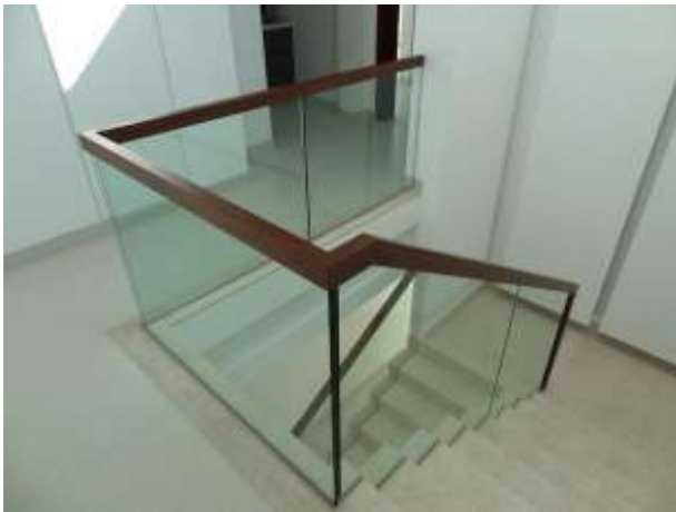
Glass & wood railing
