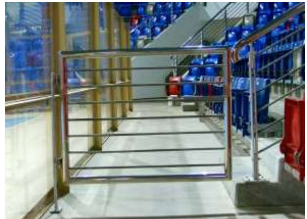
Stainless steel railing gate
