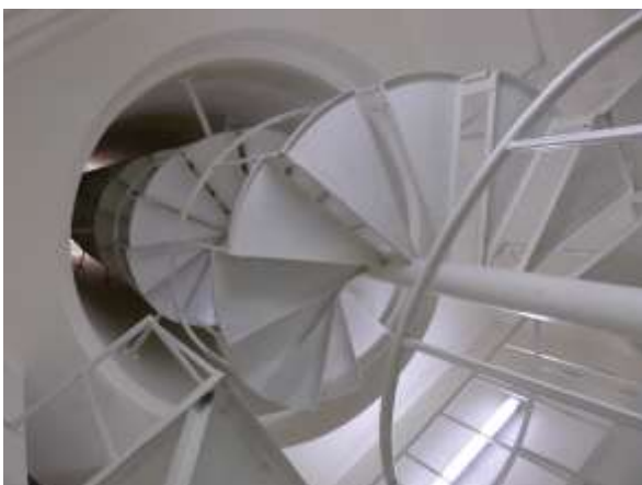
Steel spiral staircase
