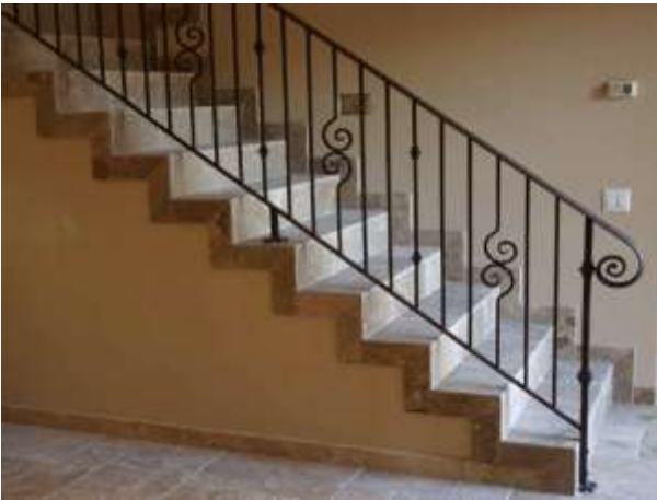
Wrought iron railing
