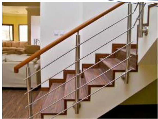
Stainless steel & wood railing
