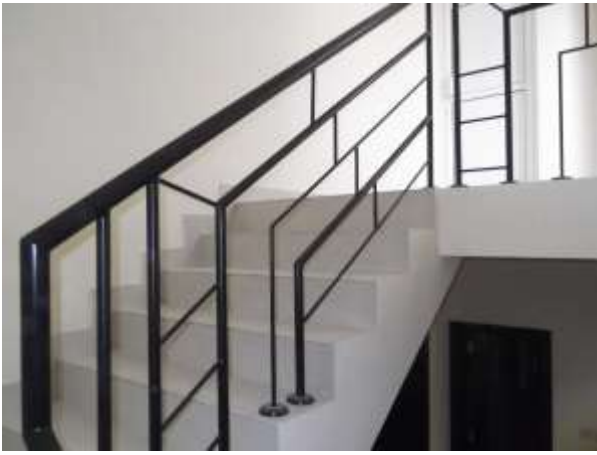
Painted steel design railing
