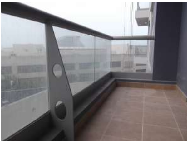
Aluminium and glass railing
