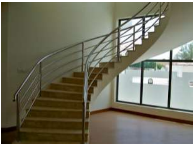
Stainless steel curved railing
