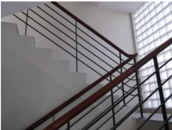
Steel and wood railing
